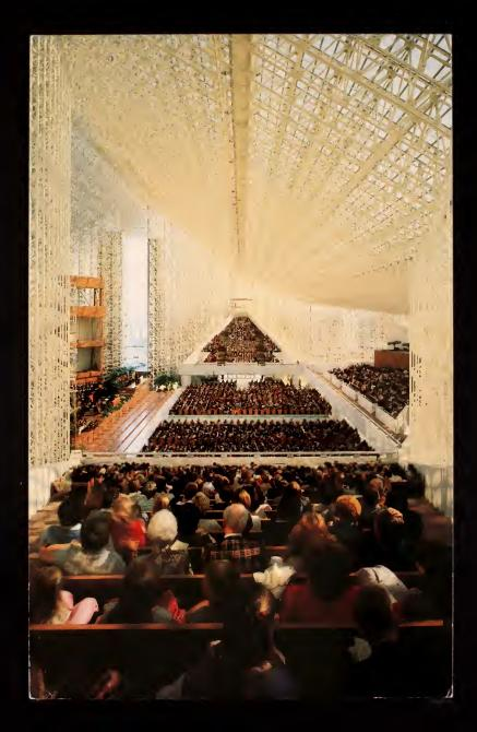
The interior of the Crystal Cathedral, Garden Grove, CA. The white, steel trusses form a lace-like frame to hold 11,400 windows. 90 foot doors open to minister to drive-in worshipers. From point to point, the Cathedral spans a full 420 feet, with seating capacity of 2,862.
